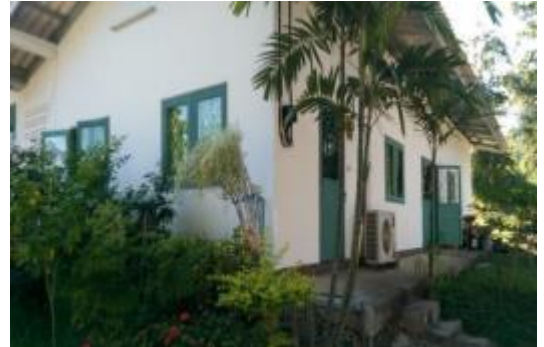
Fig 3. Repairing cutting room (Oct-Nov 16).
