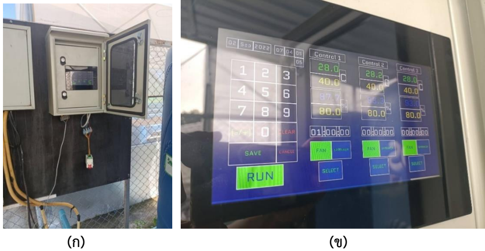
Figure 6.1-4 Development of the environmental control cabinet (a) The developed environmental control cabinet to control the fan and humidification pump. Time can be set accordingly. (b) Improved HMI screen.
