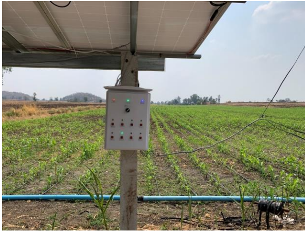
Figure 3 Installation and commissioning of the smart watering control system.
