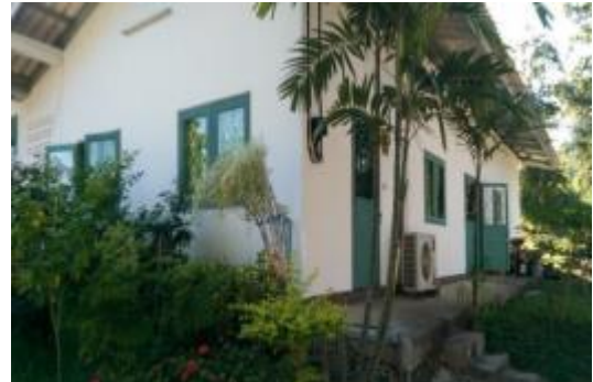
Fig 3. Repairing cutting room (Oct-Nov 16).
